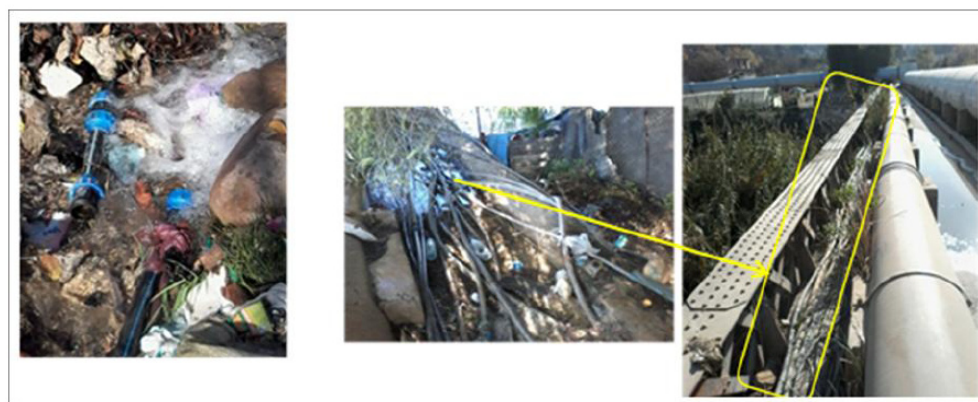
Figure 5. Illegal connection to a drinking water network –Stage 12 (Field Investigation, 2017)
