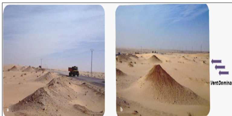
Figure 12. the immediate approach of the road is completely desilted and the effectiveness of the cone method on the national road RN 16 (Tougourt to El Oued) (Source: C.R.S.T.R.A, 2015)
