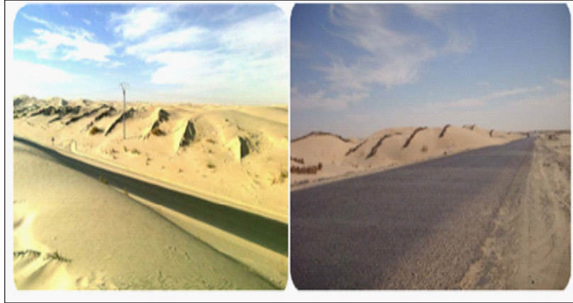
Figure 13. Successive palisades laid perpendicular to the direction of the prevailing wind (Robbah-Oued) (Source: author, 2022), the photo on the right represents palisades based on palms laid obliquely to the road to be protected (El Oued-Robbah) (Source: C.R.S.T.R.A, 2015).
