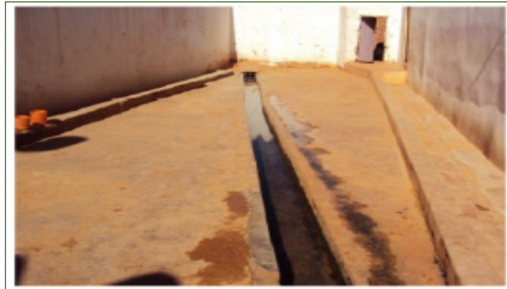
Figure 7. View of the seguias of hourly foggara in Timimoun. [Authors, 2022]
