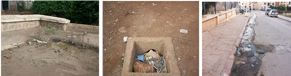
Figure 11. Poorly maintained drains with accumulated waste (source : Authors, 2022)
