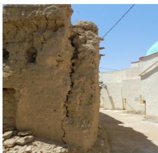
Figure 30. a). Passing crack due to differential settlement. Sabre stroke (Ksar de khanguet sisi nadji). b). Inter-intermediate differential settlement. (Ksar of khanguetsidinadji). c). The removal of mud bricks. (Ksar of khanguet sisi nadji).
