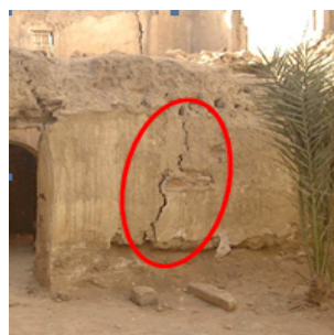
Figure 30. a). Passing crack due to differential settlement. Sabre stroke (Ksar de khanguet sisi nadji). b). Inter-intermediate differential settlement. (Ksar of khanguetsidinadji). c). The removal of mud bricks. (Ksar of khanguet sisi nadji).
