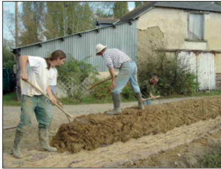
Figure 3. construction of a wall in bauge.
