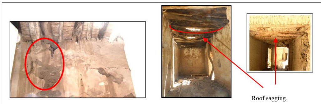
Figure 24. Trace of condensation with water run-off because of the bad junction of the beams and the wall. (Ksar of khanguet sidi nadji). Source: Author:2022.
