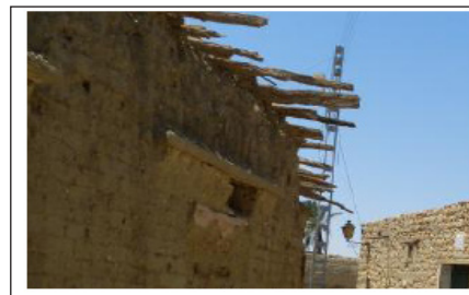
Deterioration of structural wood due to poor embedding
