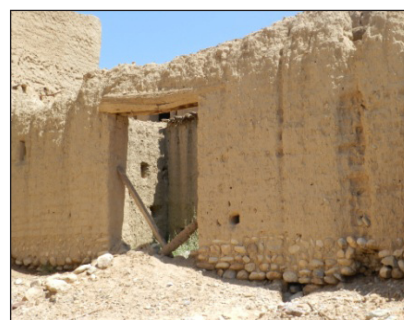
Figure 19. Erosion of the bottom of the wall in a building in the ksar of khanguet sidi nadjî. Source : Author.2022.
