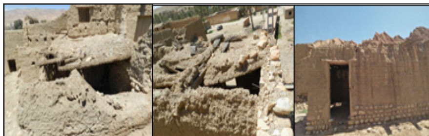
Figure 26. Degradation of the wall - detachment of the plaster of the interior space and the façade - erosion of the head of the wall. (Ksar of Khanguet Sidi Nadji). Source : Author 2022.
