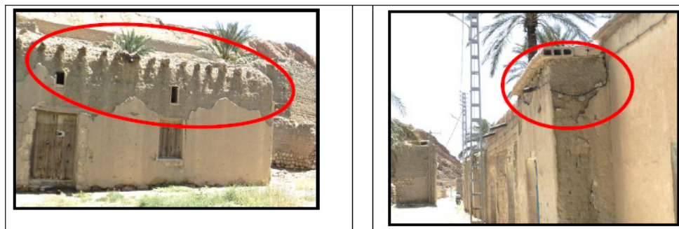
Figure 31. Detachment of the plaster due to the use of waterproofing materials unsuited to the properties of the adobe. (Ksar of khanguet sidi nadji). Source : Author.2022
