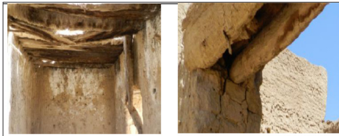
Figure 28. Deterioration of palm wood due to water retention. (Ksar of khanguet sisi nadji).
