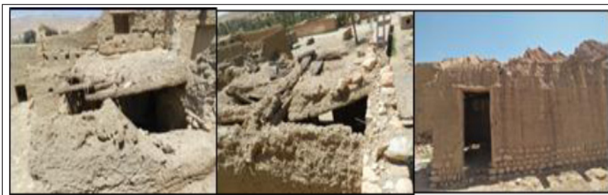
Figure 27. Degradation of the roofs of the houses due to the retention of rainwater. (Ksar of khanguet sidi nadji). Source : Author:2022
