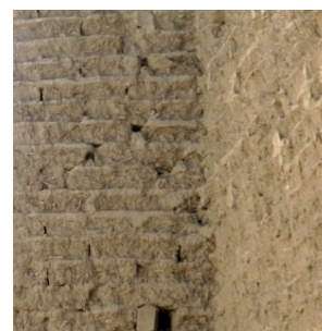
Figure 30. a). Passing crack due to differential settlement. Sabre stroke (Ksar de khanguet sisi nadji). b). Inter-intermediate differential settlement. (Ksar of khanguetsidinadji). c). The removal of mud bricks. (Ksar of khanguet sisi nadji).
