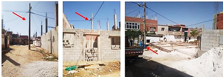
Figure 6. Medium voltage power lines encroach on roadways and densely populated areas (Source: Authors, 2022)
