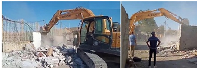
Figure 4. Demolition operation (Source: Enasr Journal, 2014)
