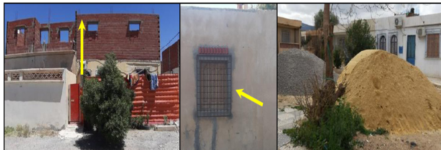
Figure 15. Vertical and horizontal expansion, Created new windows, and Putting building materials on the road when building workshops are opened (Photos taken: March 2021).
