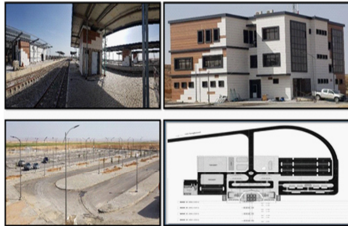
Figure 4. plan and photo of the station, Source: official documents, photos taken by the author
