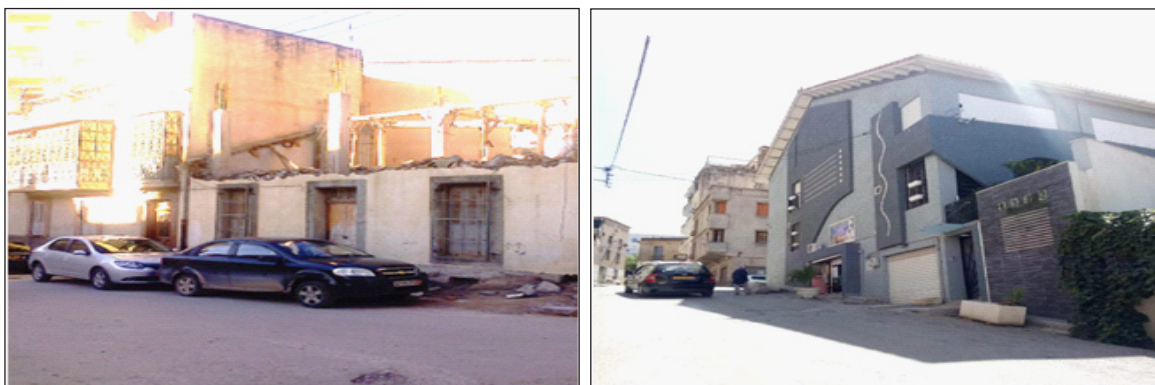
Figure 2. Mutations across the downtown, Demolition of an old building, and reconstruction of a new, more modern one, Source, Bensakhria 2016 and 2022
